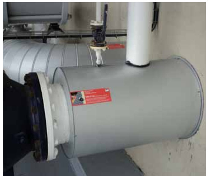
Fire resistance for fire-wall pipe penetrations
