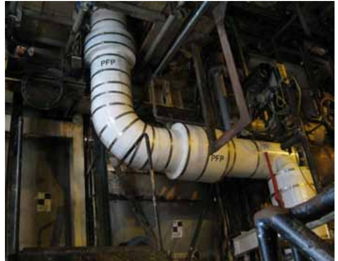
FOAMGLAS® XP: up to two hours of jet-fire resistance
