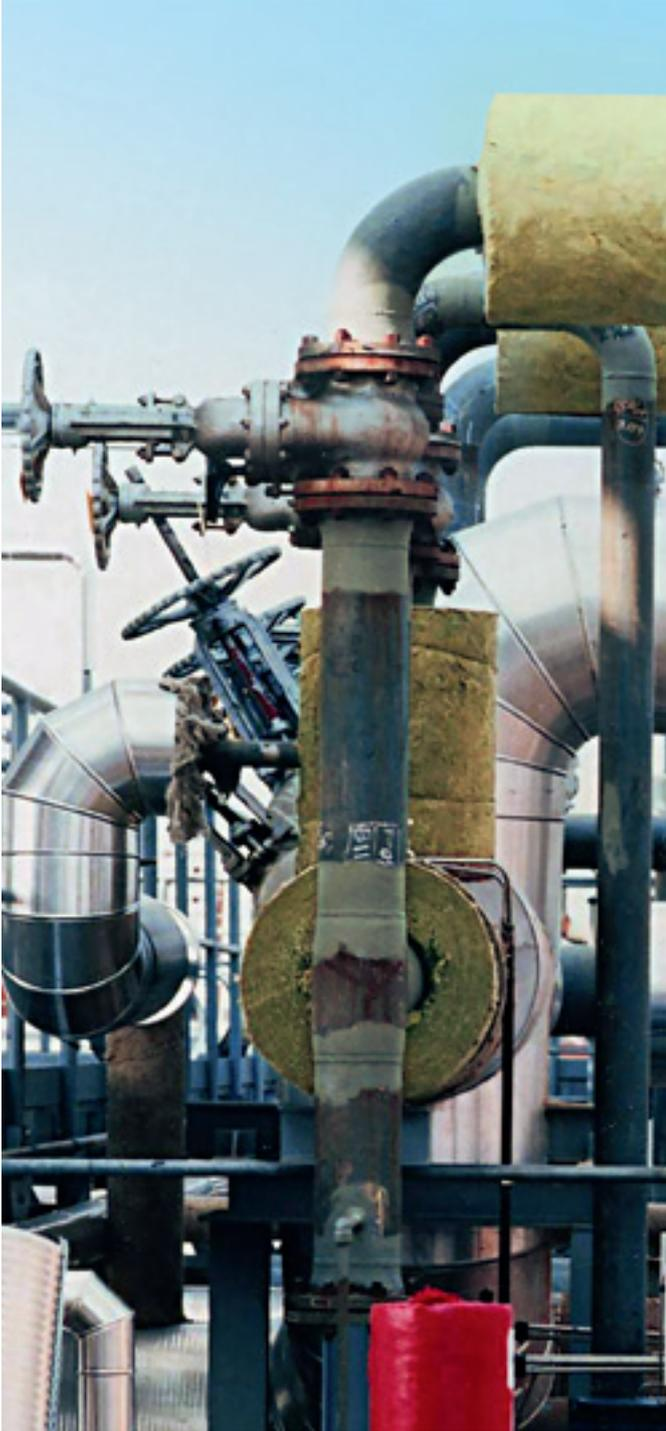
Corrosion Under Insulation (CUI) refers to the external corrosion of piping or equipment that occurs underneath externally cladded insulation due to water or moisture penetration.
