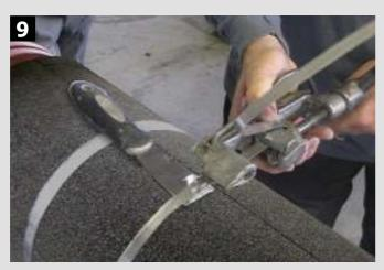
FOAMGLAS® Insulation can also be secured with stainless steel fixing straps.
