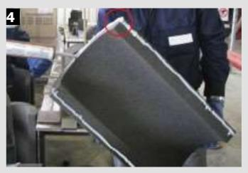
Apply PITTSEAL<sup>®</sup> 444N out of a caulking cartridge with an extrusion gun in beads to one of the jointing edges of a pipe shell.
