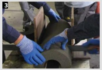
Use a hard-point hand saw to cut the  $\mathsf{FOAMGLAS}^{\circledast}$  insulation on site.
