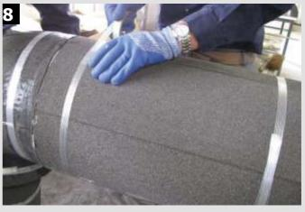
FOAMGLAS® Insulation should be secured with self-adhesive glass fibre reinforced tape.
