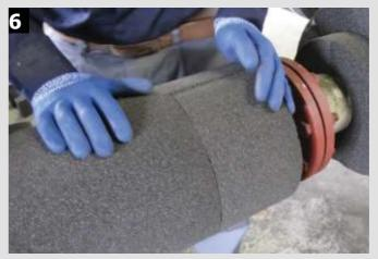
Divide a 600 mm pipe shell into pieces of 150, 300 and 450 mm and use the different lengths to stagger the joints.
