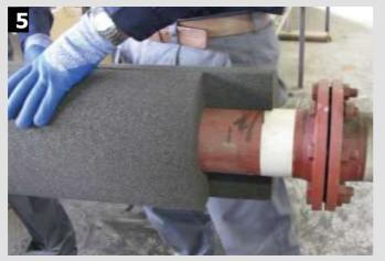
All pipe shells must be installed with staggered joints.
