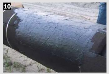
For outdoor piping that could be subjected to temperatures below the freezing point, Pittsburgh Corning's Pittcote<sup>®</sup> 300 cell filler is recommended.
