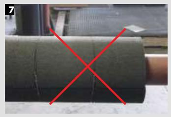
Never use wire to fix FOAMGLAS® insulation shells or segments, due to the fact that wire wil cut the FOAMGLAS® insulation surface.
