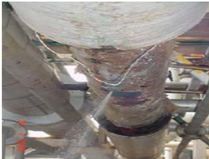
The extreme result of water penetration, product escapes!
