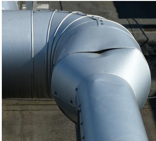
External application - The result of foot traffic and no inspection and maintenance!
