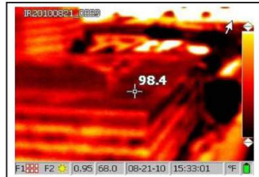
Metal drain cover
