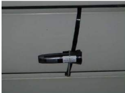
Typical Data Logger installation
