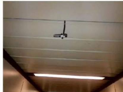
Bridge Data Logger
