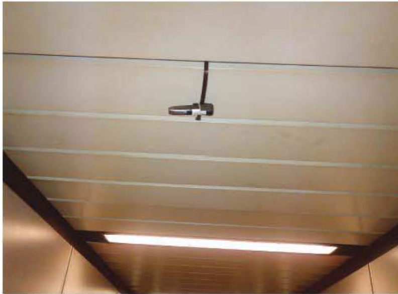
Dry bulb thermometer inside the bridge
