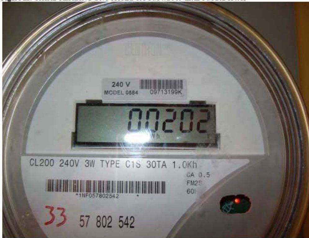
Figure 12: THIRD READING UNCOATED ROOM 7/14/09 12:13 PM 202 KWH
