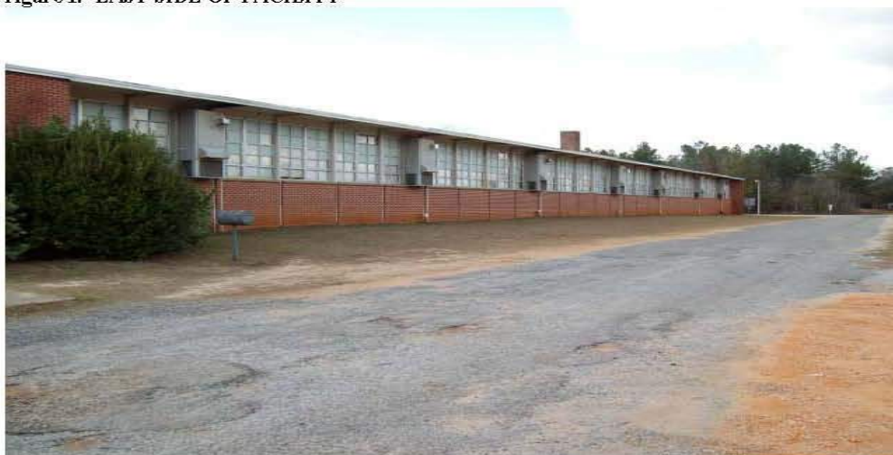
Figure 1: EAST SIDE OF FACILITY
