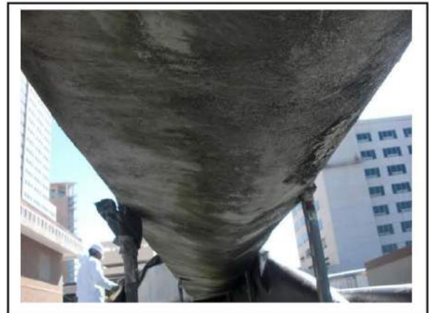
Bottom of duct has insulation that is bellied out with water
