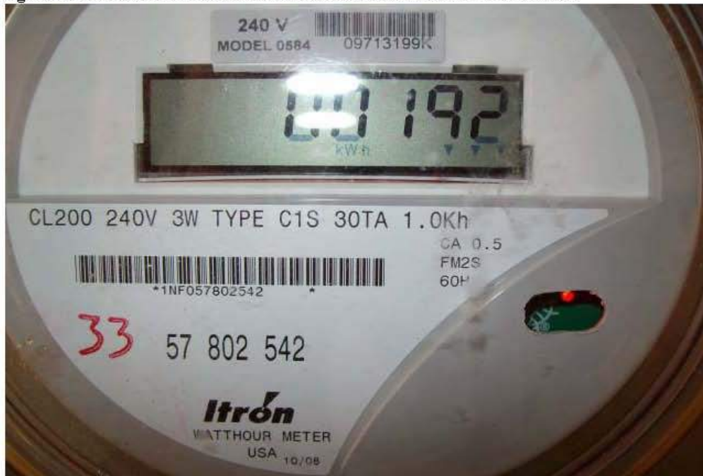
Figure 10: SECOND READING UNCOATED ROOM 7/13/09 2:58 PM – 192 KWH
